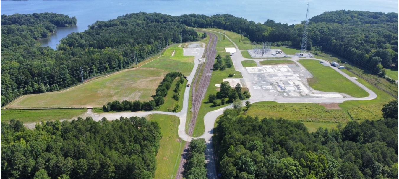
Mecklenburg Power Station, Clarksville, Virginia, July 2023.
